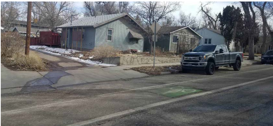
Existing bike lane in the Casper Area
