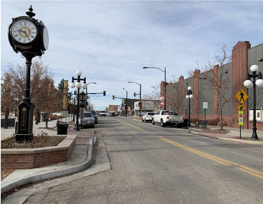
Midblock curb extensions at David Street Station
